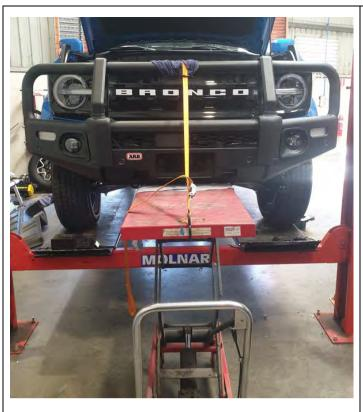
82. Using two people or a lift table, lift the bumper up to the vehicle. On the initial fitment, it is recommended to use two of the chassis mount spacers. If you have a winch, the control box may contact the plastic. (Ignore it for the time being, it will be trimmed later).
